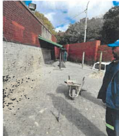
After – work in progress
