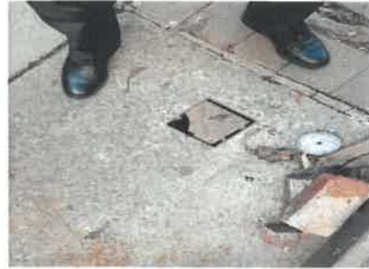
After – leak fixed
