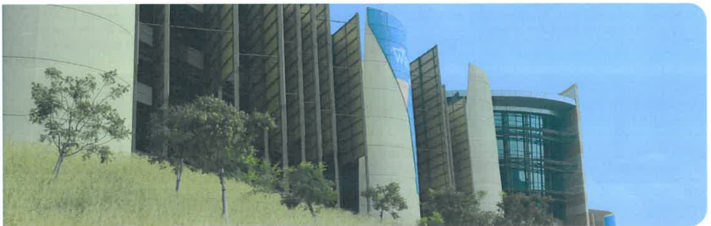
Metro Centre Street View
