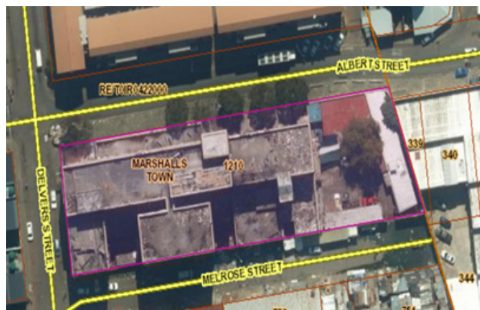
Figure 13: Usindiso Block – Marshalltown
